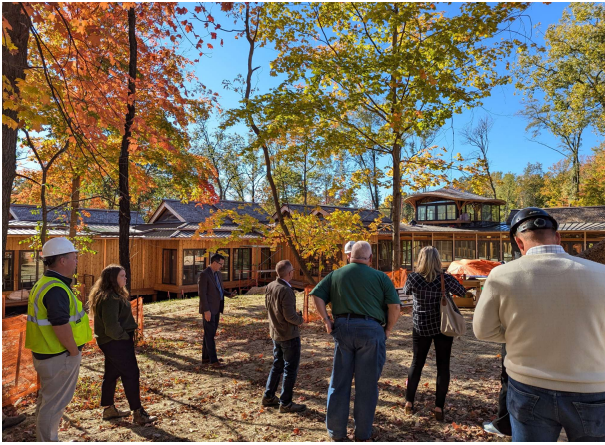
Ongoing construction at the JST site on 12 Mile Road
