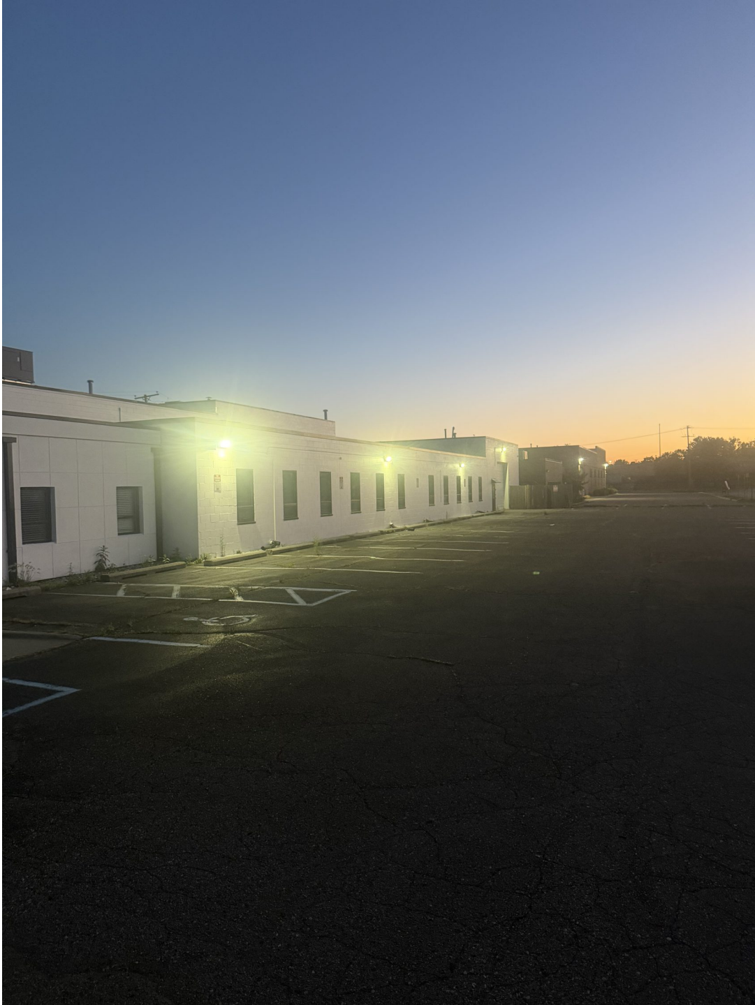
Photo 4 — South elevation, full building length
