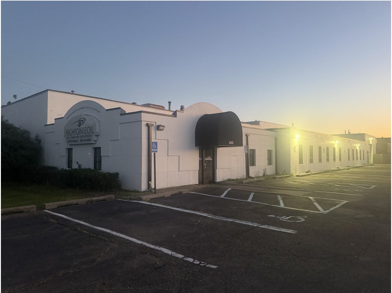
Photo 2 — Main entrance and northwest corner
