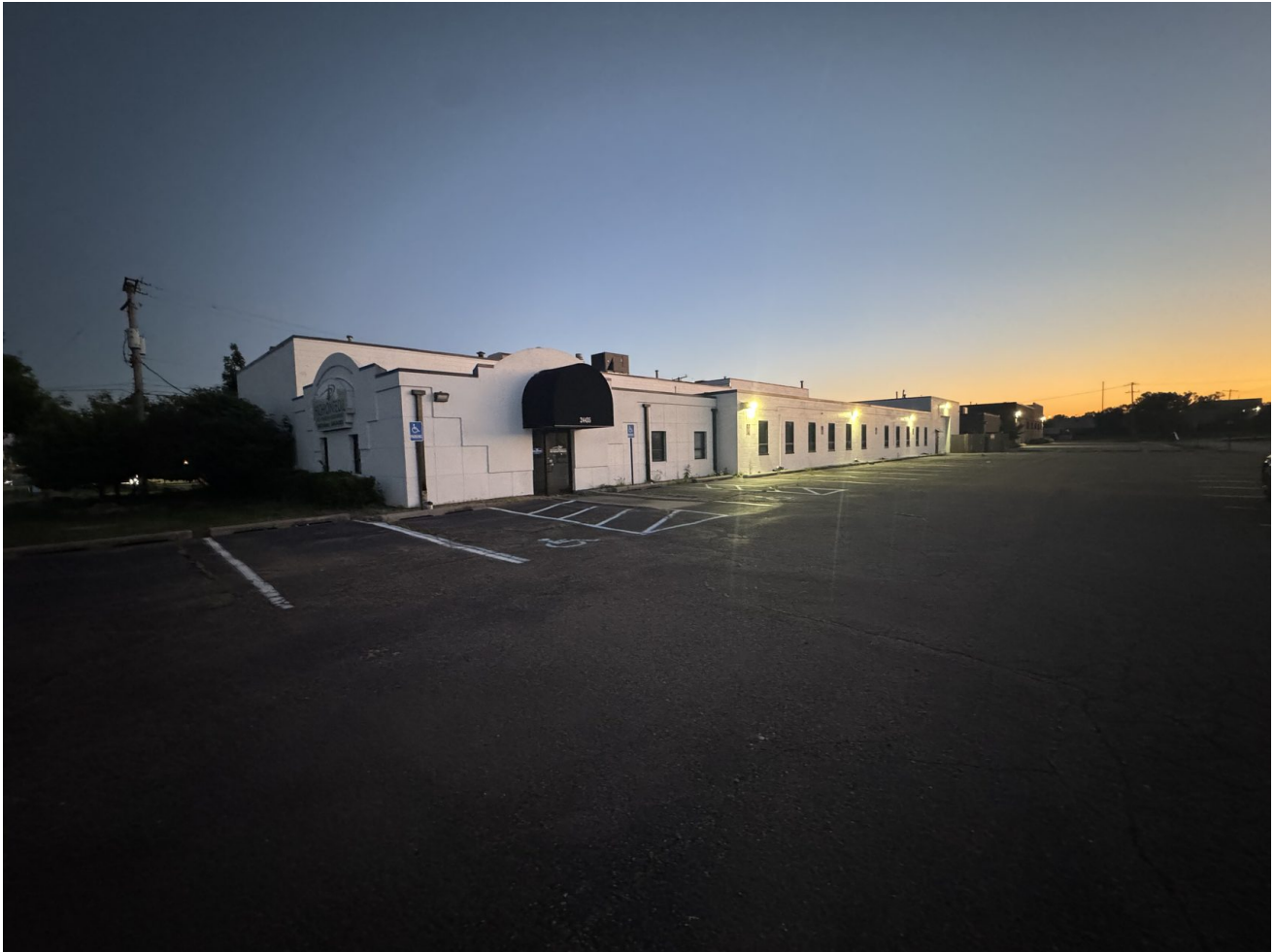
Photo 3 — South elevation, fixture spacing
