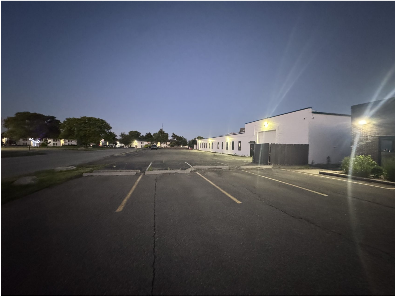
Photo 7 — Overall site illumination at night
