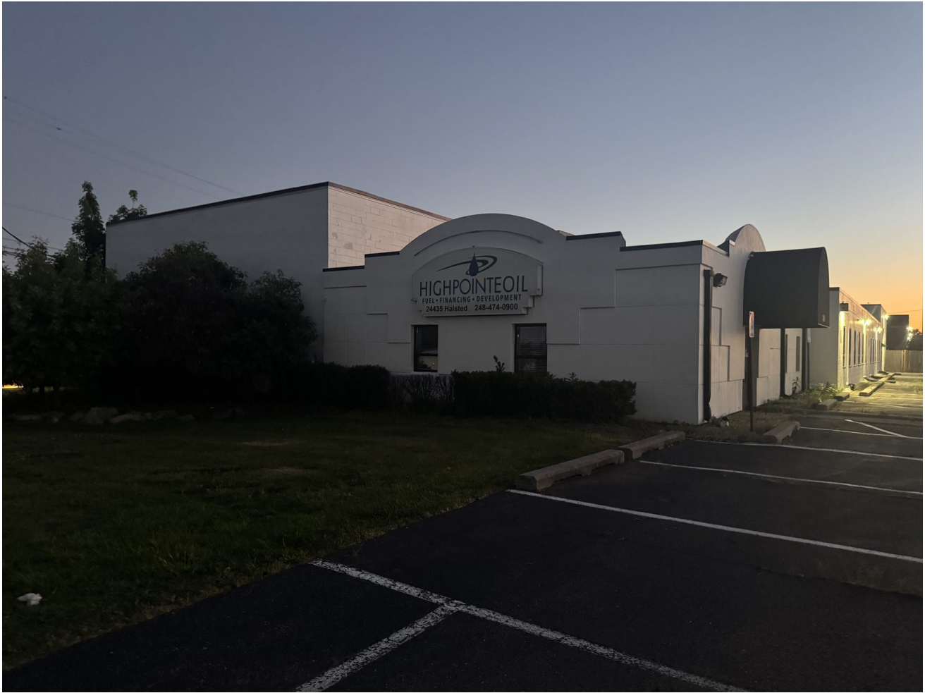
Photo 1 — Front (Halsted Road) elevation
