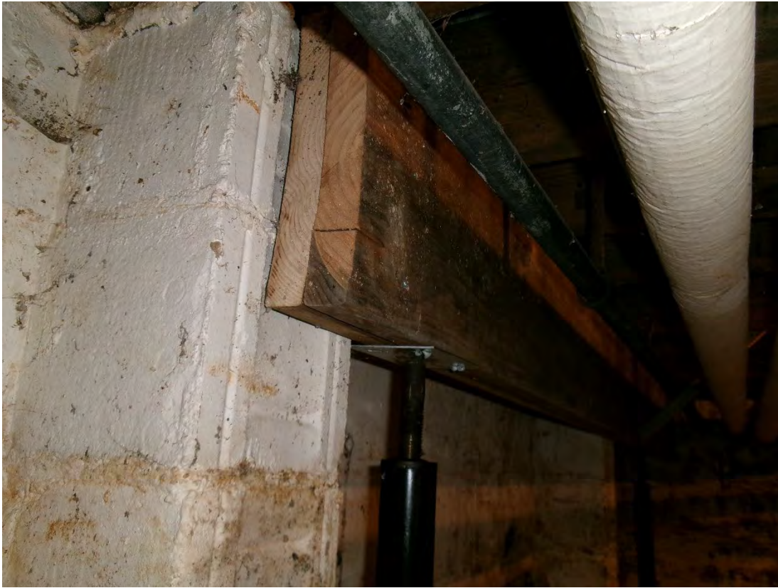
Basement floor jack supports
