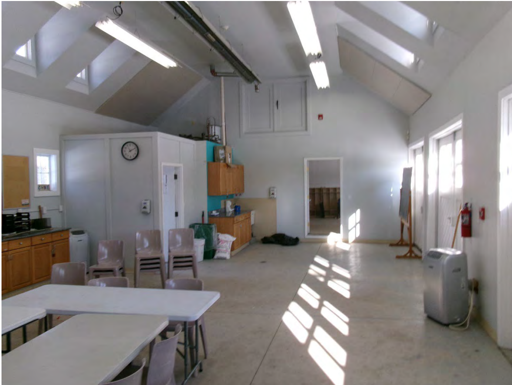
6e6 Egress doors, exit signs and emergency lighting
