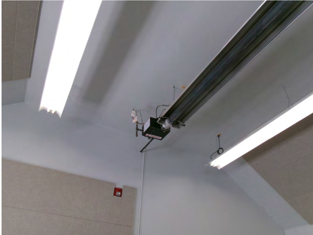
6e5 Gas fired radiant heater
