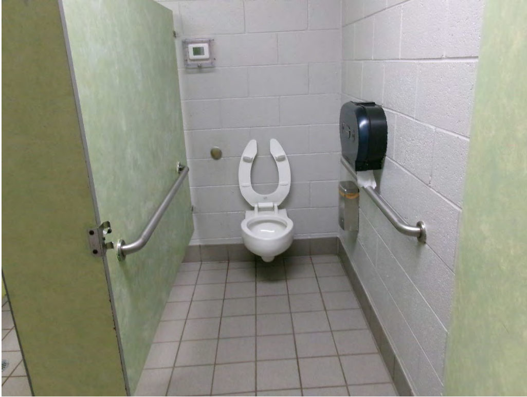
9d3 Women's ADA toilet
