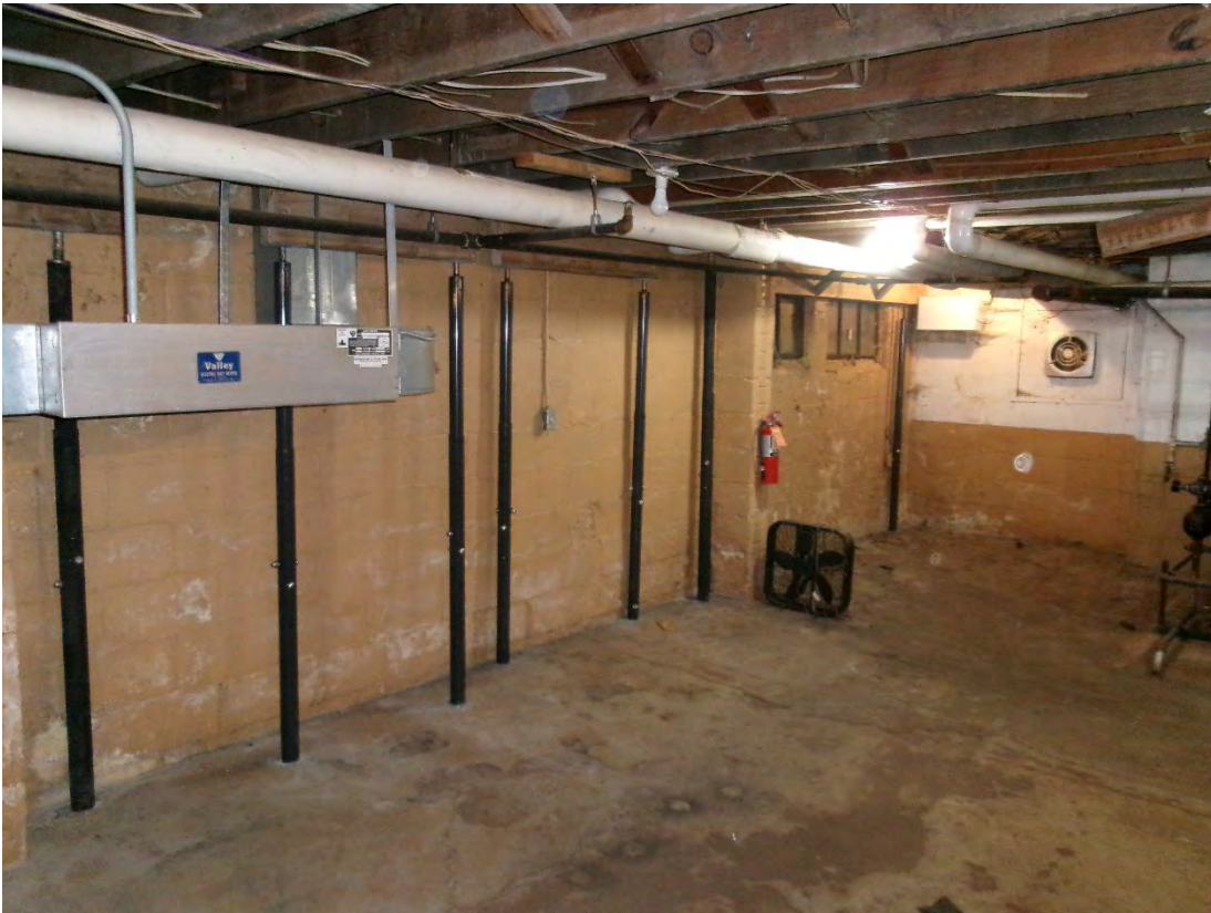
Basement floor jack supports
