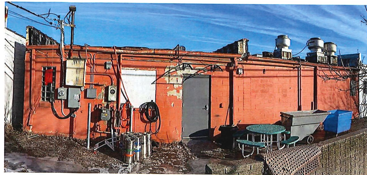
3 EXISTING CONDITIONS VIEW SCALE: NONE
