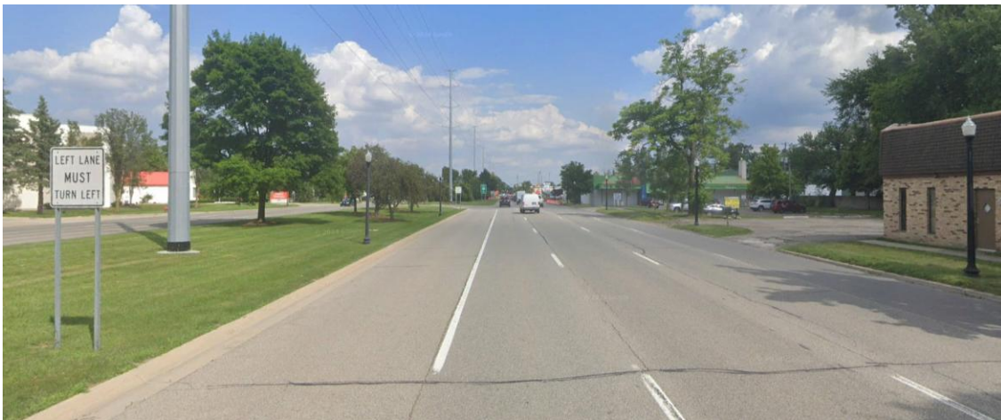
Figure 24: Grand River Avenue looking south toward 8 Mile Road.
