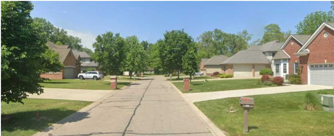
Figure 19: Kimberly Court neighborhood located northeast of 8 mile and Tuck Roads
