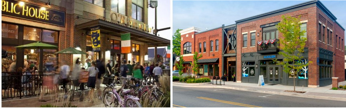
Figure 10: A small neighborhood mixed-use village would offer the Grand River neighborhoods and businesses an attractive live, work, and shopping destination. Left, Eddie Street, South Bend, IN, Right Ada, MI new villages.
