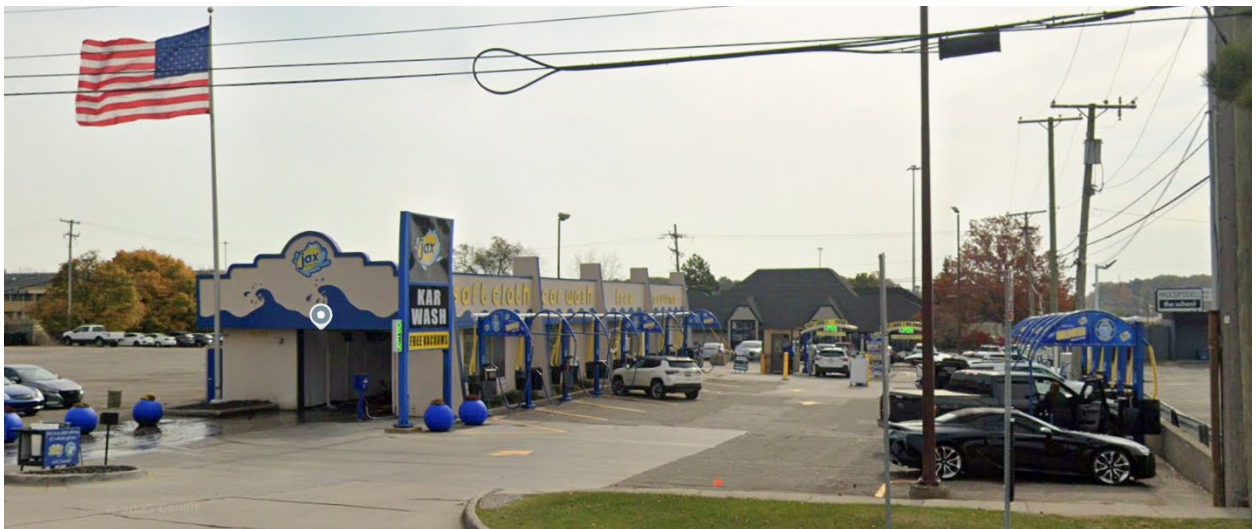
Figure 2. View of north and west elevation fronting W 12 Mile Rd (view towards south).
